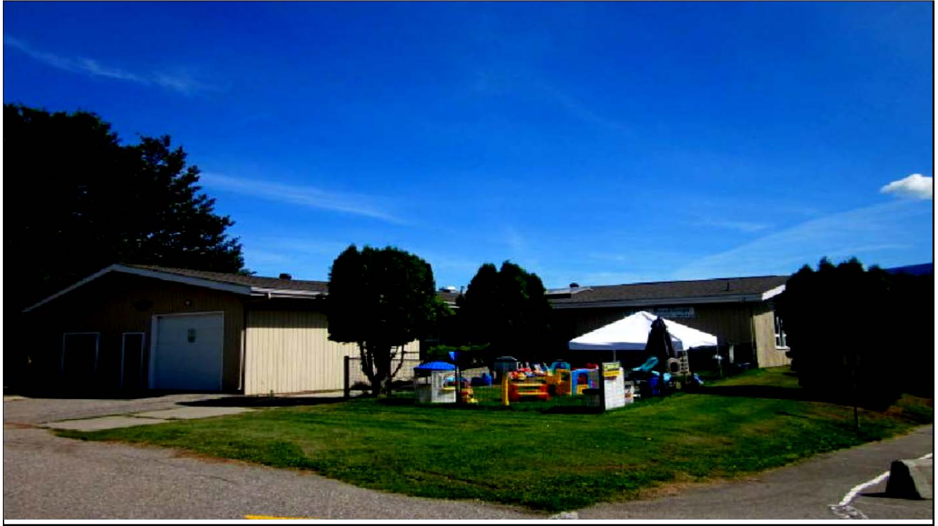
Photo of Facility
