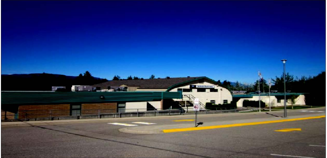
Photo of Facility
