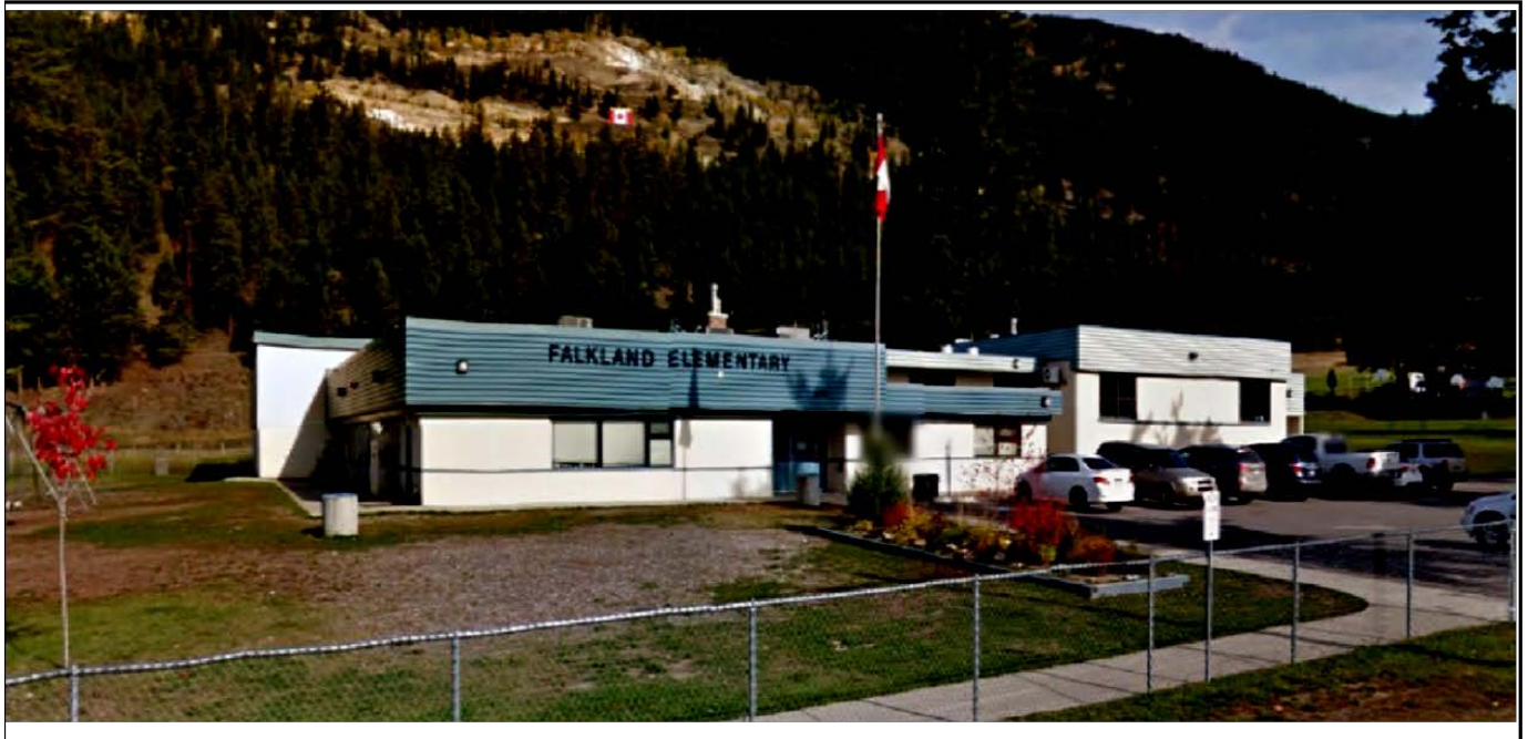
Photo of Facility
