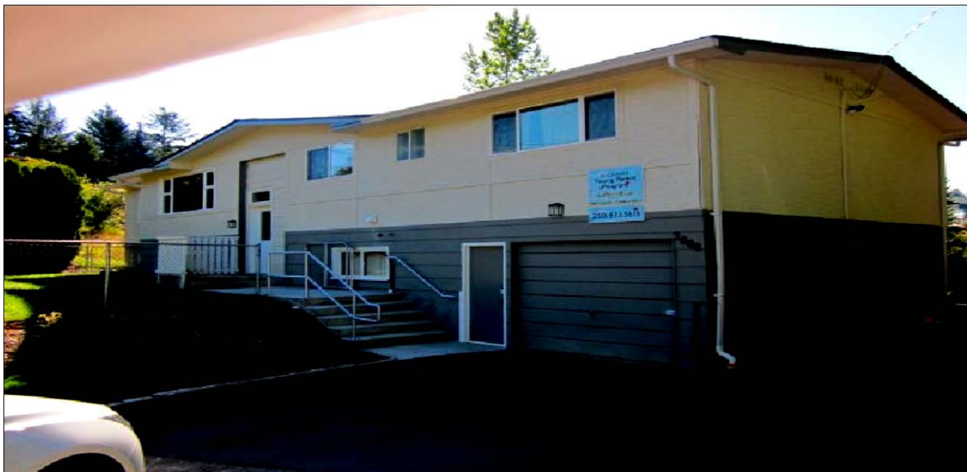
Photo of Facility
