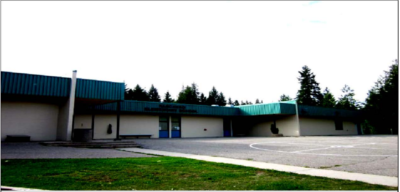
Photo of Facility
