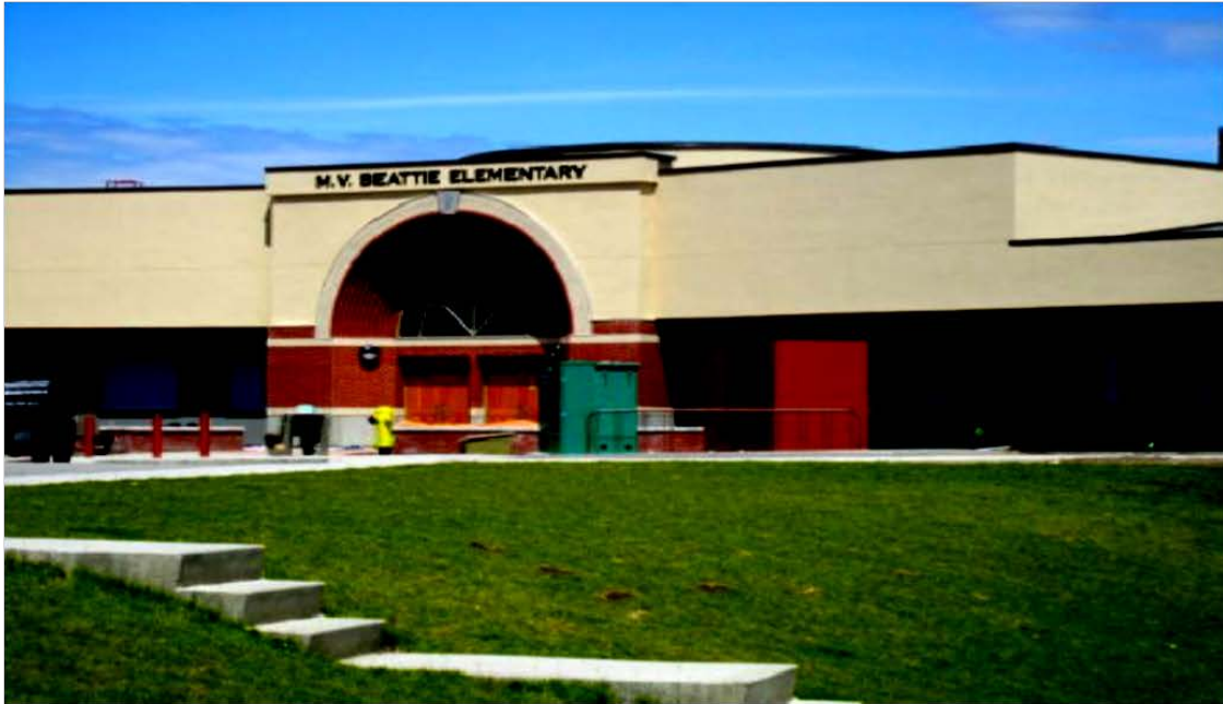
Photo of Facility
