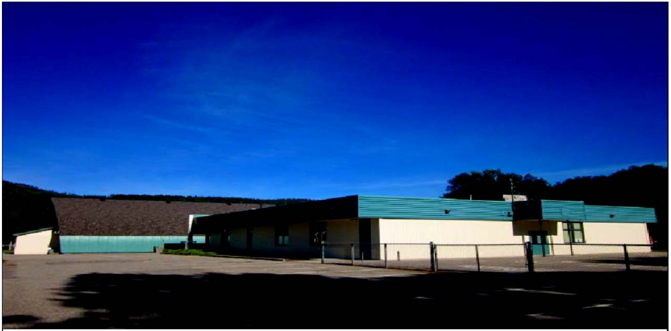
Photo of Facility
